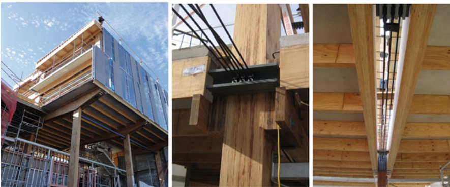
Fig. 13.30 College of Creating Arts – MacDiarmid Building, Massey University, Wellington, New Zealand. Post-tensioned timber (Pres-Lam) frames in the transverse directions with horizontal U-Shape flexural plate dissipaters on the first floor and Post-tensioned concrete (PRESS) walls in the longitudinal direction (Structural Engineers: Dunning Thornton Consultants)
