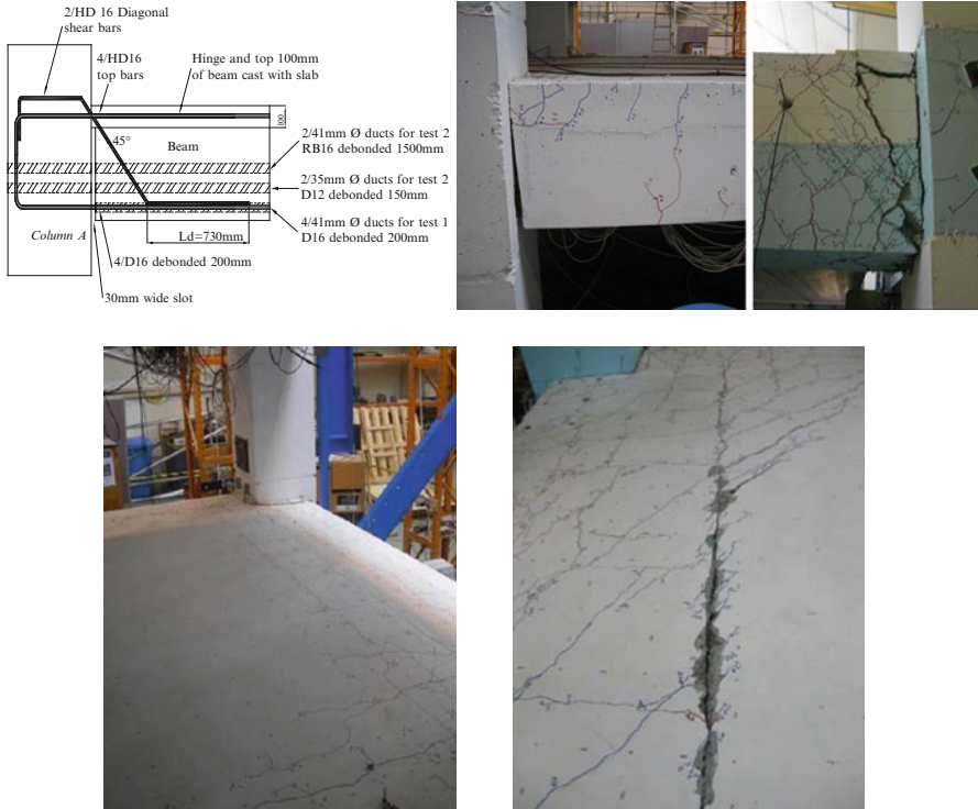
Fig. 13.17 “Non tearing floor” or top-hinge solution: Top left : schematic (left, Muir et al. 2013) and comparison of damage to plastic hinges ( Top centre and right ) and to the floor ( bottom left and right ) from the testing of a 3-D superassemblage implementing a top-hinge solution ( top centre and bottom left , Muir et al. 2012) vs. a traditional beam-column connection ( top right from MacPherson 2005, bottom right , Lindsay 2004)
