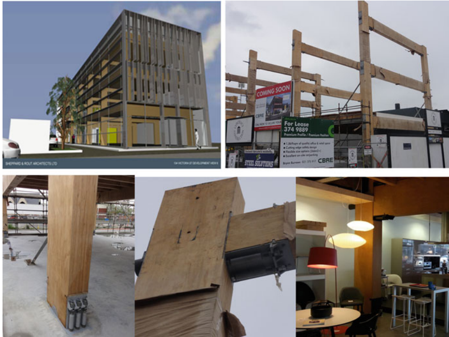
Fig. 13.31 Merritt Building, Victoria Street, Christchurch. Three Storey commercial Building consisting of Post-tensioned timber (Pres-Lam) frames in the transverse direction and cast-in-situ reinforced concrete wall in the longitudinal direction (Structural Engineers: Kirk and Roberts; Architects: Sheppard and Rout)
